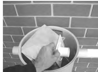
Firmly insert bag port into side of unit.
